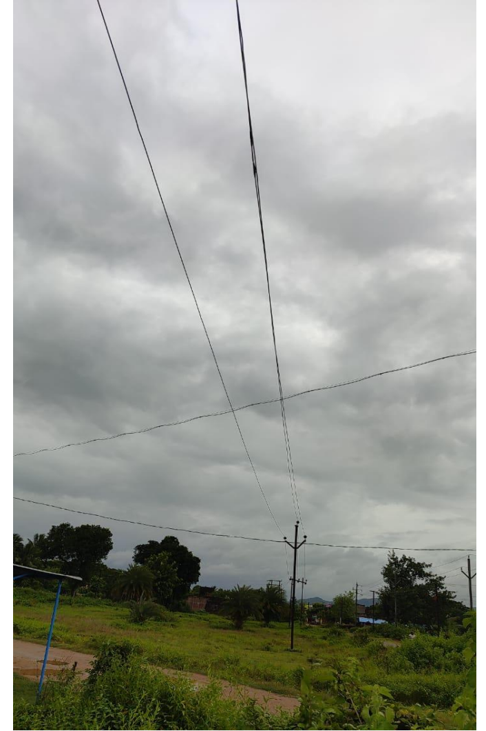
Twisted Conductor of 33KV Budhamba Feeder
